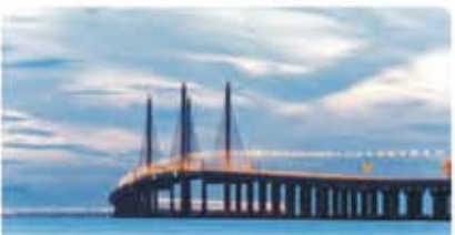
Jambatan Sultan Abdul Halim Muadzam Shah 24 km
